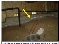
Efflorescence noted along front & side foundation walls.
