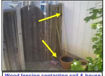
Wood fencing contacting soil & house siding.
