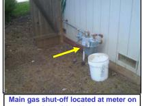
Main gas shut-off located at meter on right side of house.
